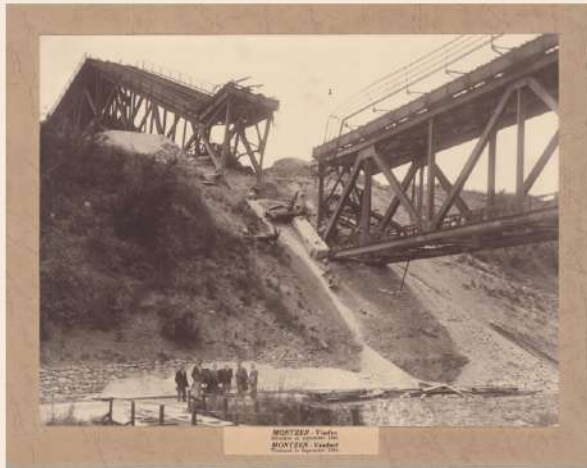
De vernielde spoorviaduct in Moresnet in september 1944
