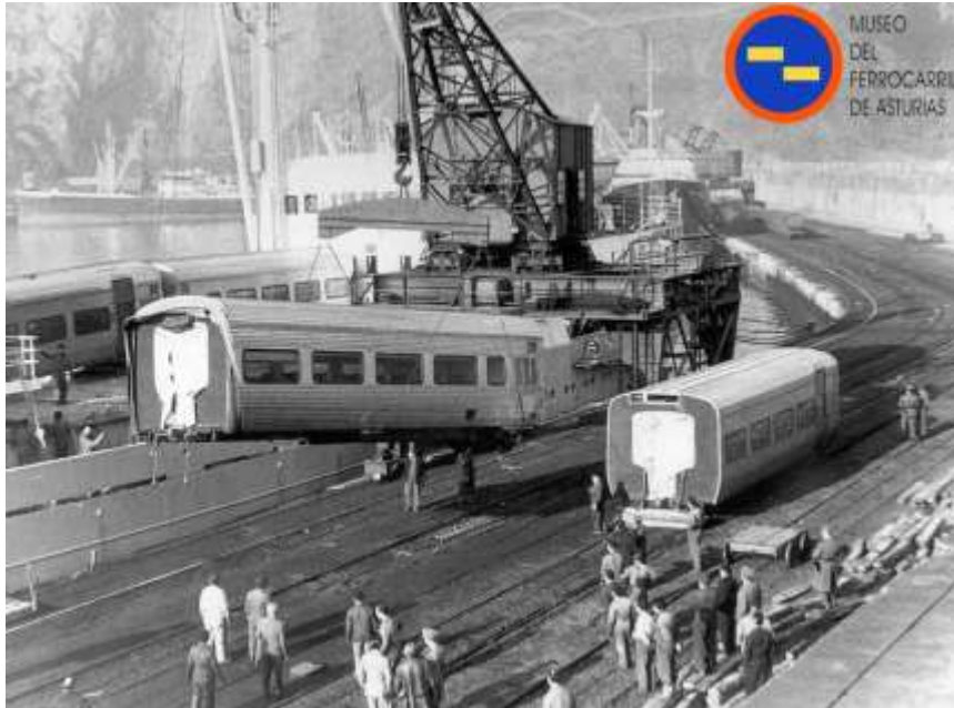
Talgo01_11 Gijon 1969. NH Talgo II cars being unloaded for use on the Langreo
