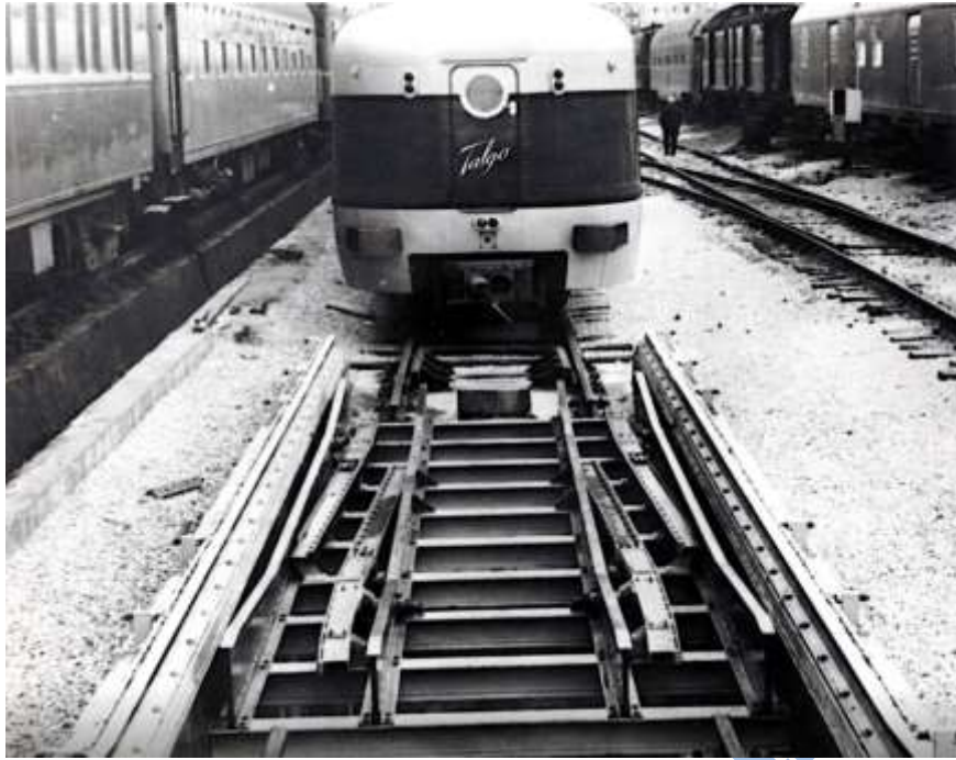
Talgo01_13 Madrid 1967. Prototype Talgo RD mechanism
