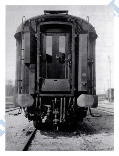
The end connectors on an unidentified steel-body car. (G.P.Keen)
