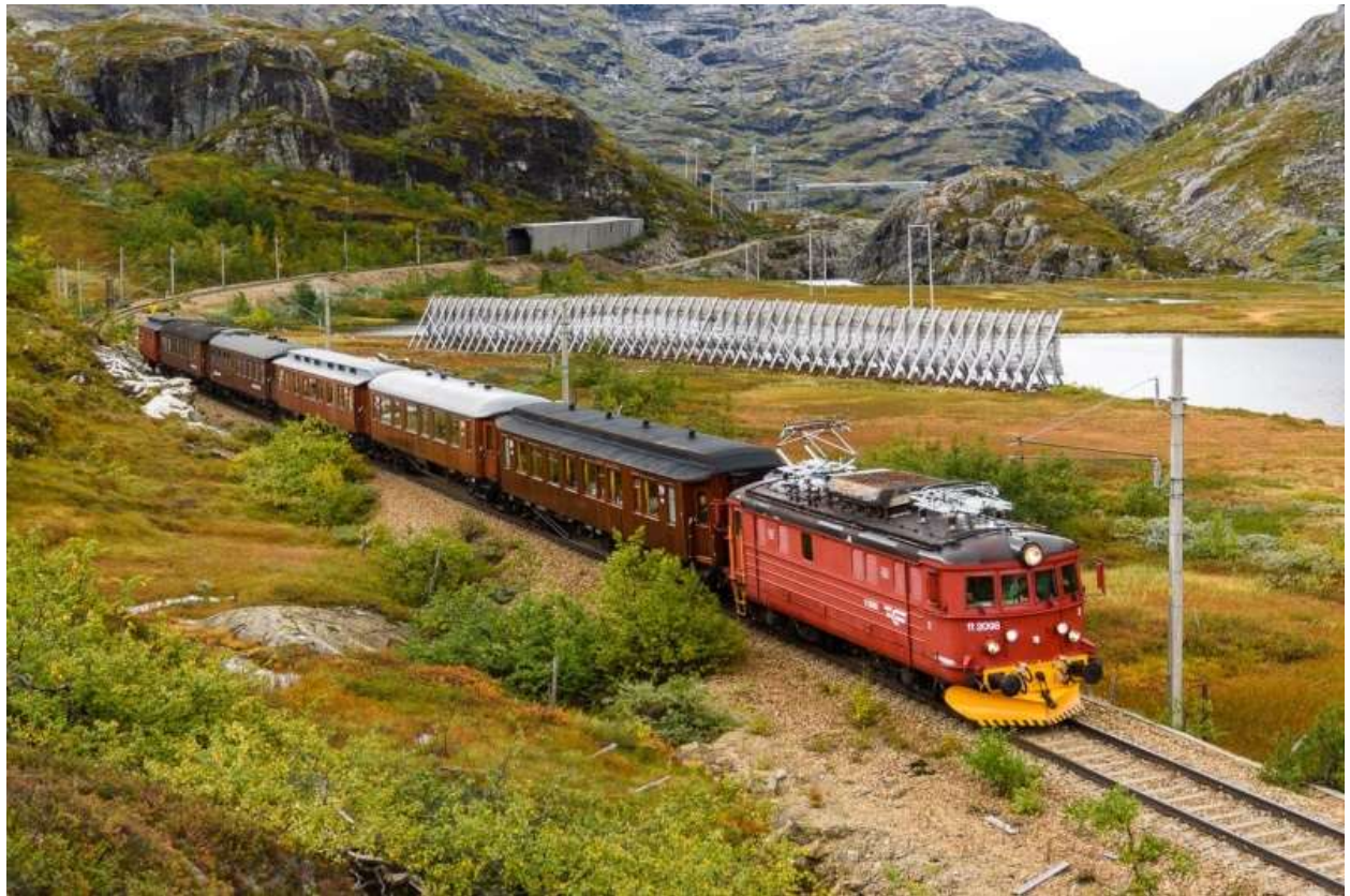
Photo 43 is taken near Myrdal on the Bergen line. Here you can see how the line is winding it's way through the landscape. The snow galleries are easy to see in the back of the train. To the left you'll also see snow fences to make the snow to stop drifting. Along the Bergen line from Myrdal to Finse there is also a single high tension power line for extra supply and security for the current of the line. Photo CF Salicath
