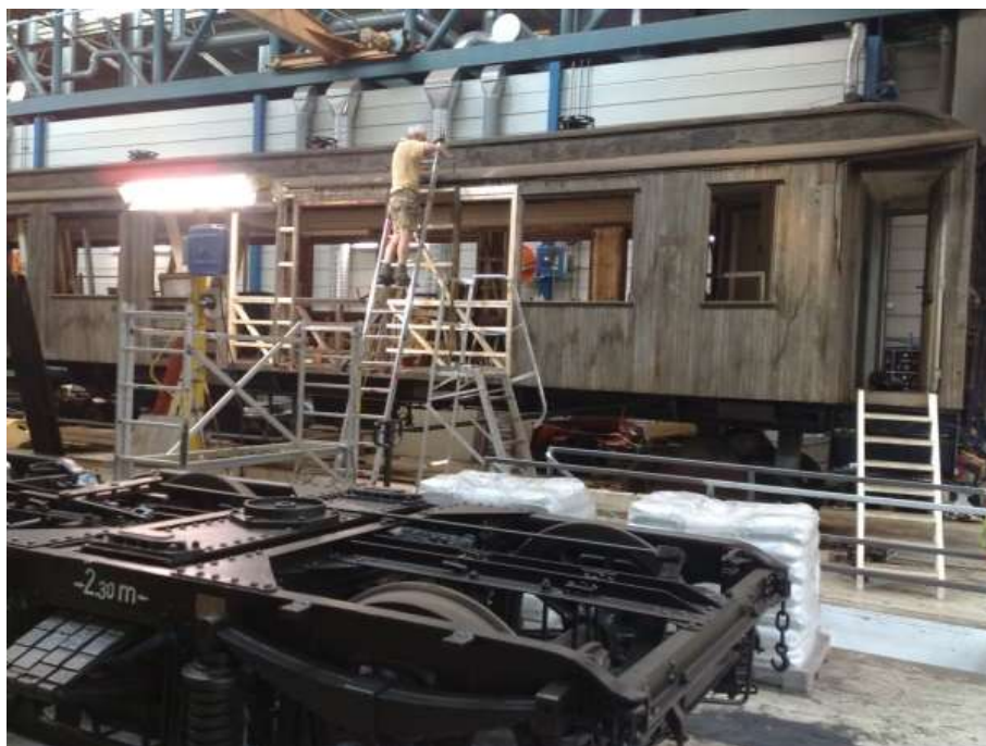
This photograph shows the coach when parts of the panelling are stripped off and we are starting to repair damage in the wooden structure. In front you can see the old bogies fully repaired and ready for new assembly.
