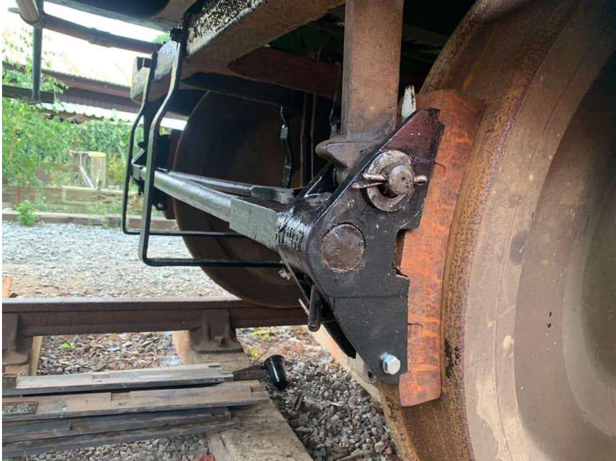
The newly restored brake rigging installed.
