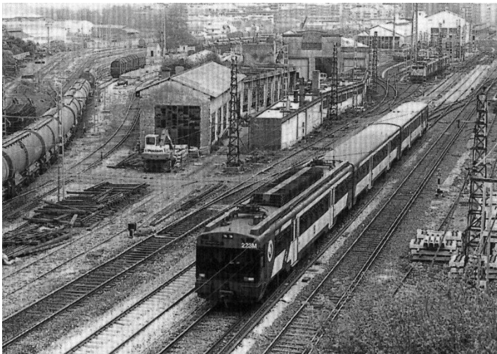
What remains of these workshops in 1998, three years after their closure. The RENFE locomotive sheds are in the background
