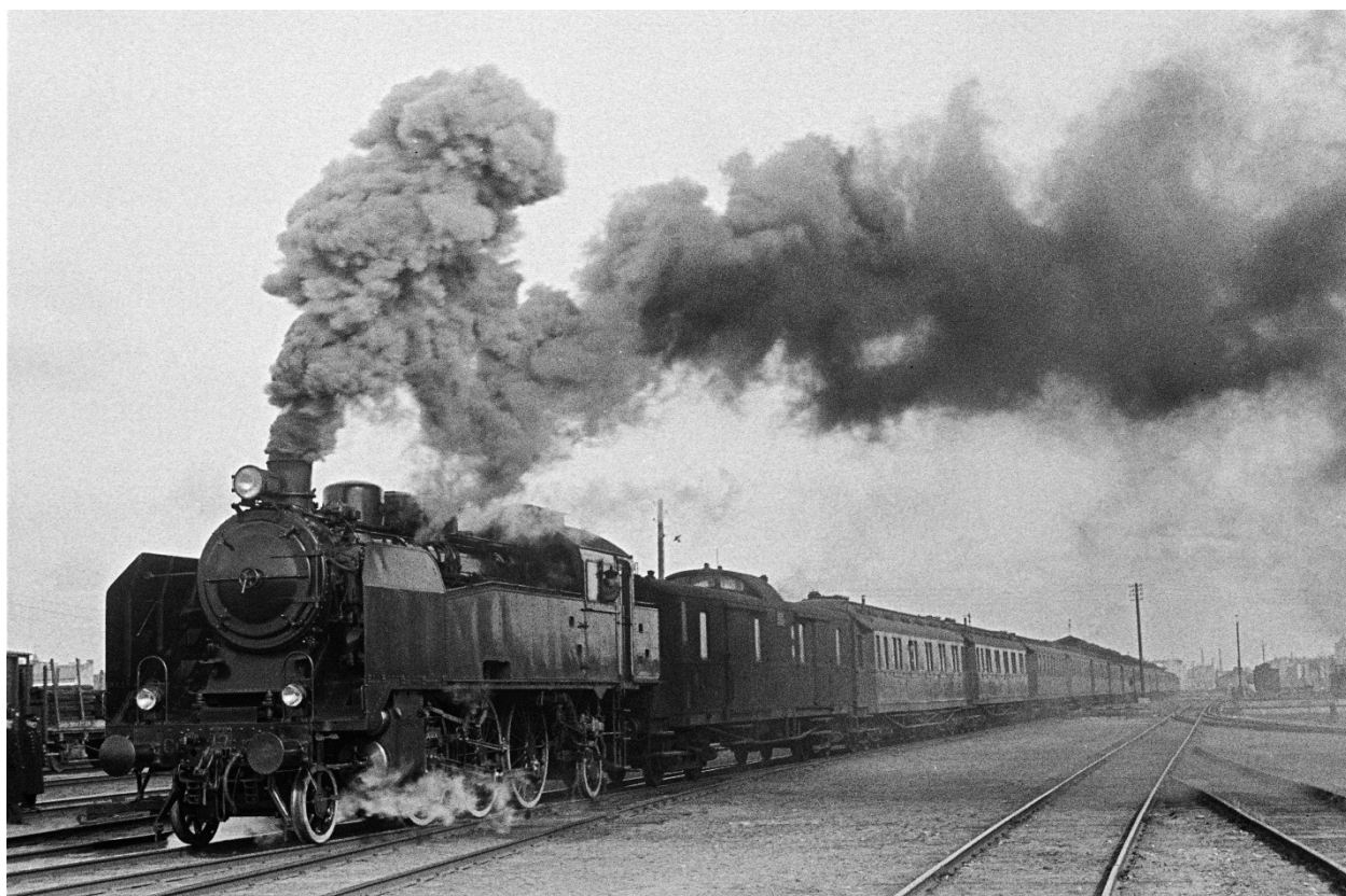
Trial run of newly built (Henschel, 1938) Ct-315 from Riga Passenger station with passenger train included two of CIWL No. 2681-2683 (ex EL 169-171), Latvian railway history museum collection.
